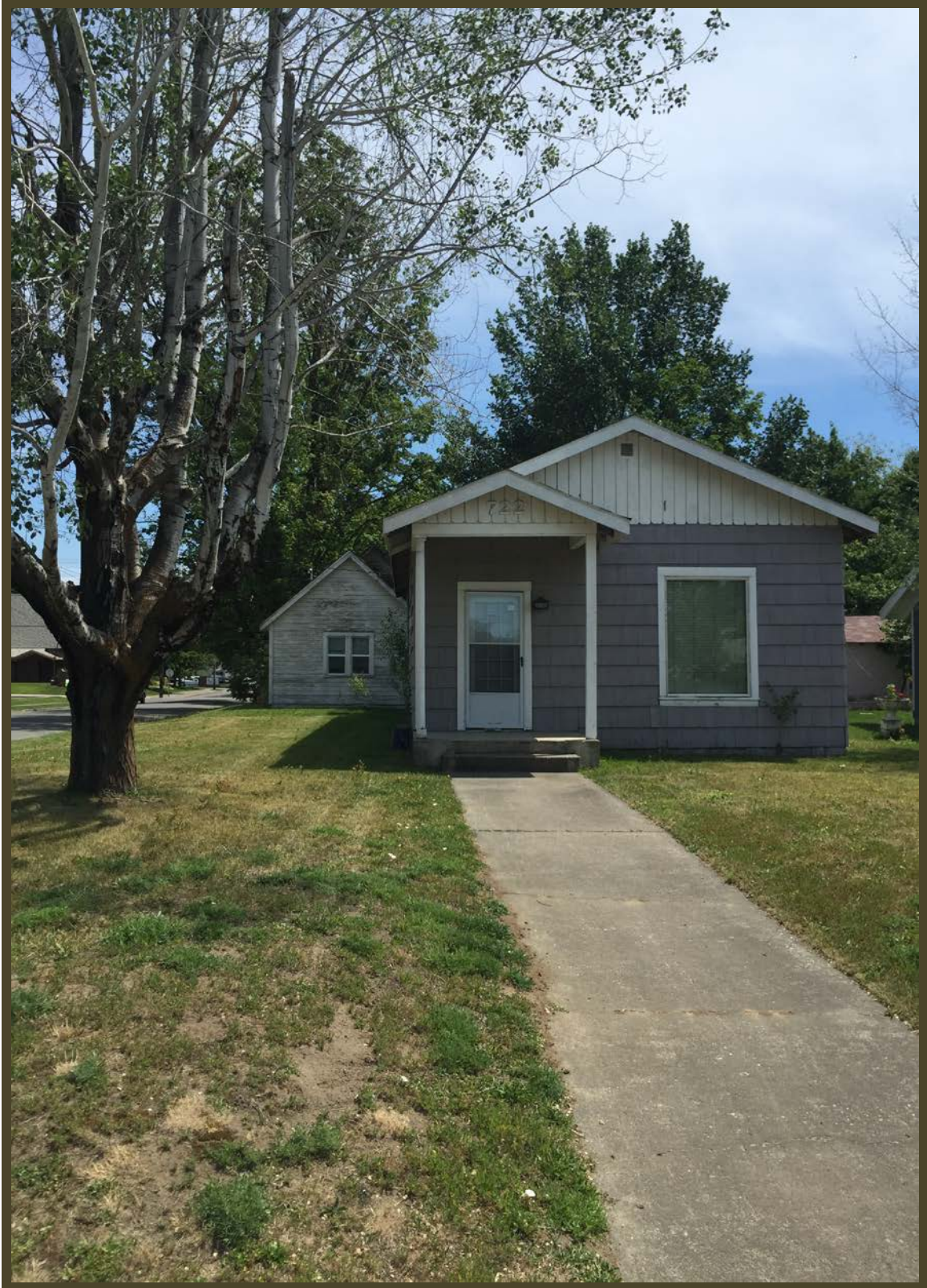
View From 4 th Street Looking East At Subject Property
