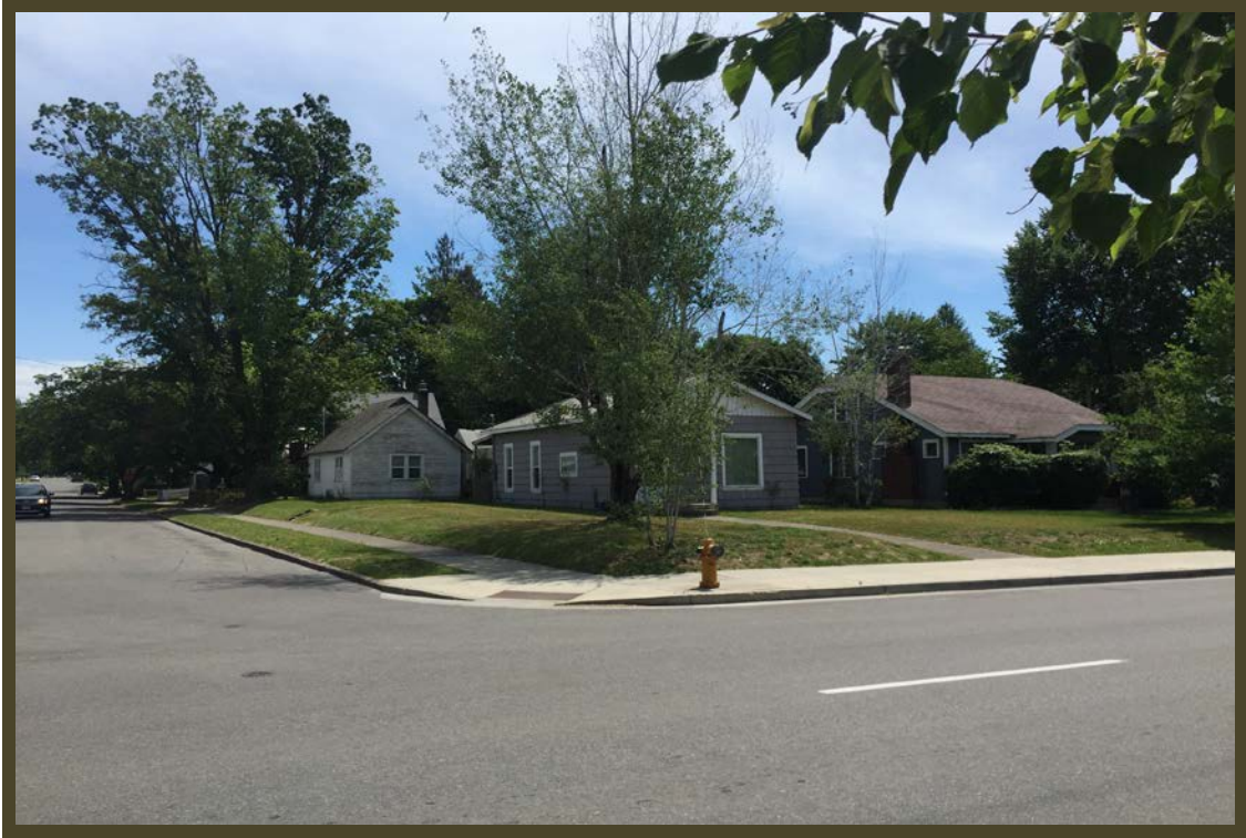
Corner View of 4 th Street & Reid Avenue Looking Southeast at Subject Property:
